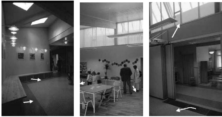
Figure 4 The ventilation air is distributed into the occupied zones via grilles in the floor or under benches (left and middle). In order to achieve efficient displacement ventilation in the classrooms, the supply air temperature is controlled to be about 19°C in the heating season, which is slightly below the room temperature set point at 20°C. The exhaust air is extracted through hatches situated about three metres above the floor (right).
