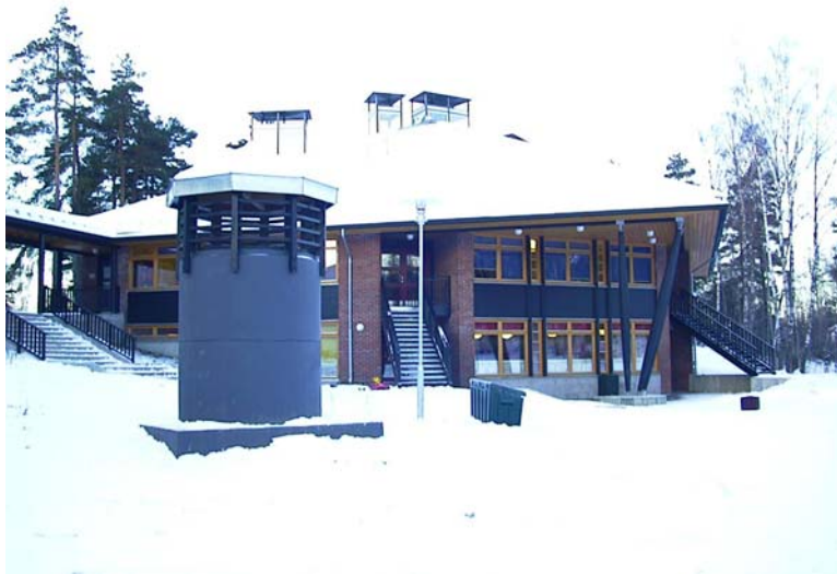
Figure 2. View of facade and air-intake tower of Jaer School, Norway
