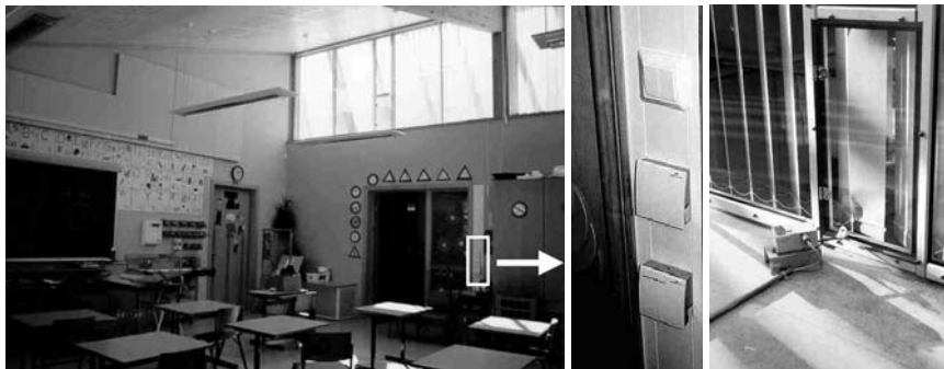
Figure 5 CO 2 sensors placed 1.2 metres above the floor level on the classroom walls (left and middle) control the opening and closing of the exhaust ventilation hatches (right) as well as the fans. Temperature sensors are placed just above the CO 2 sensors, in order to control the heating system.
